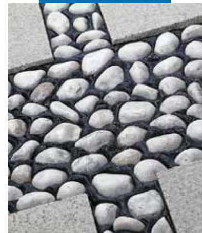
An example of grouted ornamental stones
