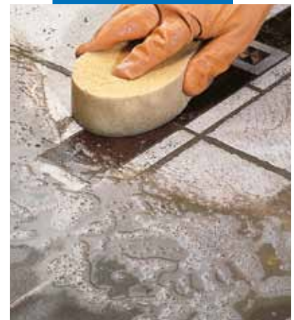
Finishing a ceramic tile floor with wood inlays with a sponge
