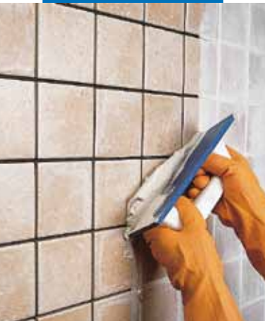
Grouting of single fired tile wall with a float
