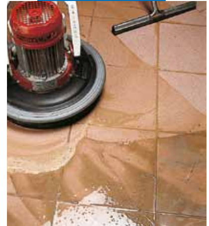
Finishing a porcelain tiled floor with single-brushed power float or rubber squeegee
