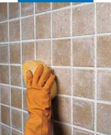
Finishing of single fired tile wall with a sponge
