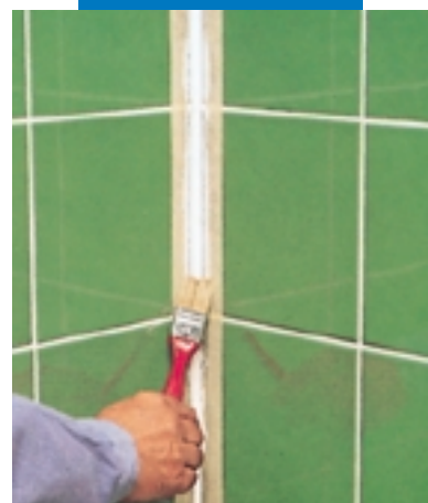
Smoothing the joint with soapy water and a small brush
