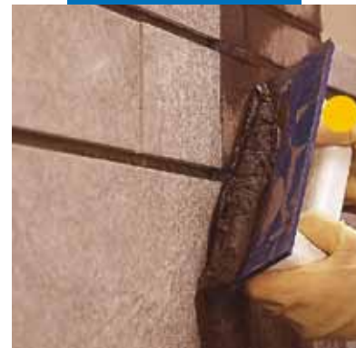
Spreading Ultracolor Plus on a wall with a rubber trowel
