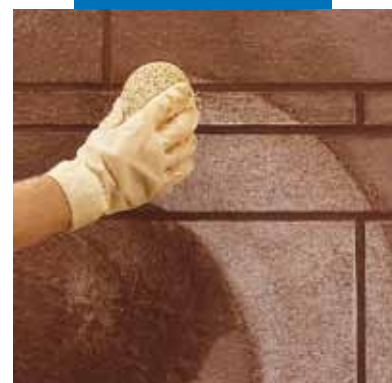
Cleaning and finishing the tile joints with a sponge
