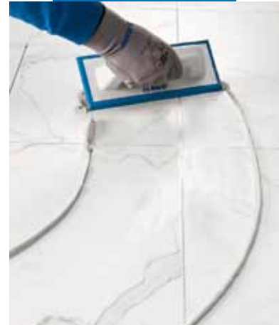
Spreading Ultracolor Plus on marble-effect porcelain floor tiles with a rubber trowel
